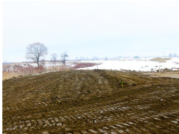
Tee area under construction
